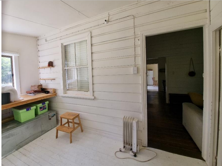
Original front wall and one original double hung 4 pane sash window within the enclosed verandah. This window provides detail for future restoration of the replaced windows.
