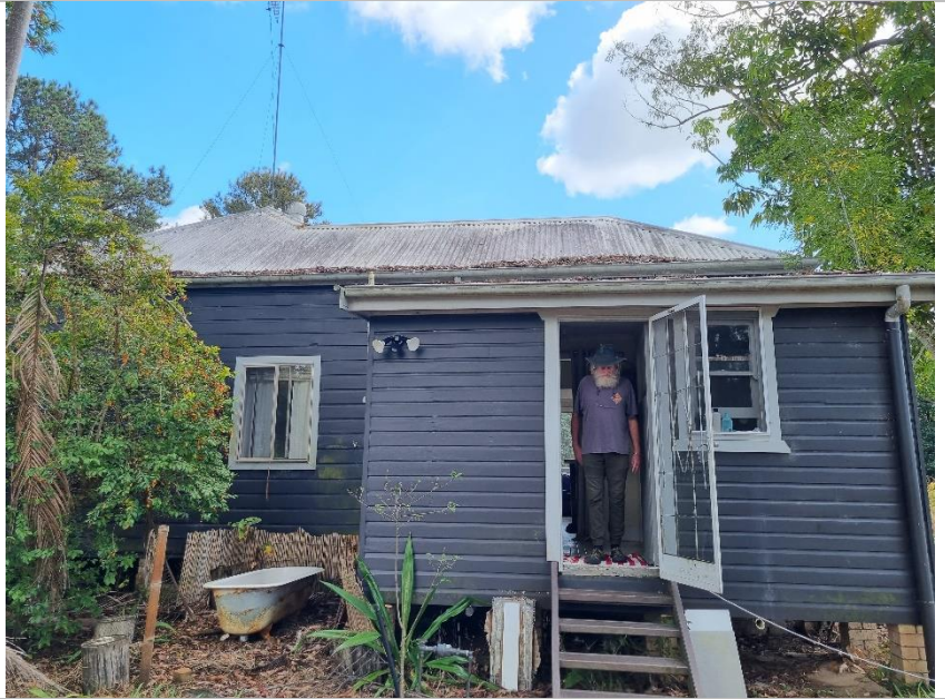
Southern side elevation and skillion roof addition at rear.
